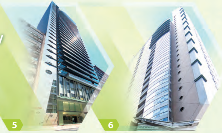
5 Trendy Centre 6 Prosperity Center Property (portion)
